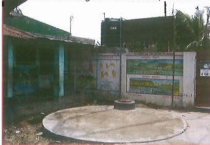
Rainwater Harvesting at Suravi School, Baniabadh
