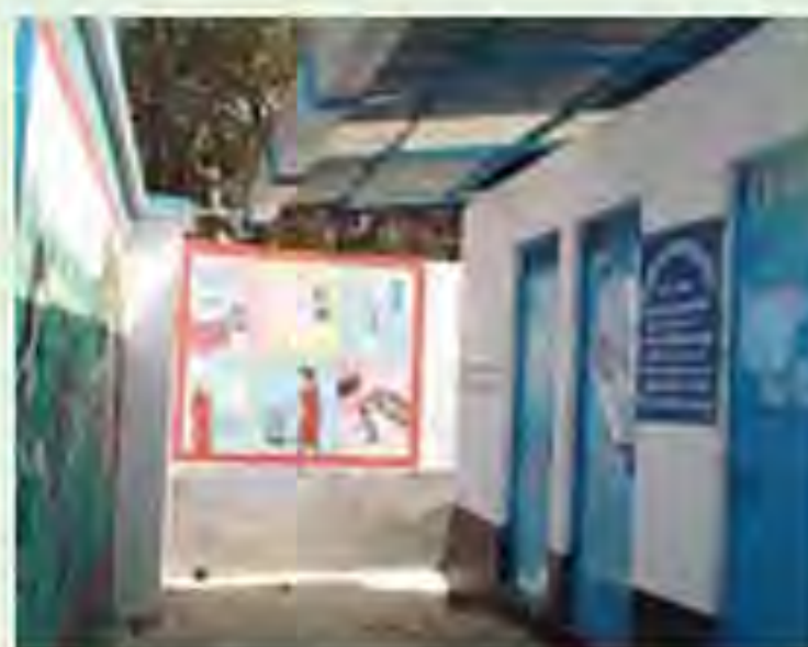
Renovated Toilet at School
