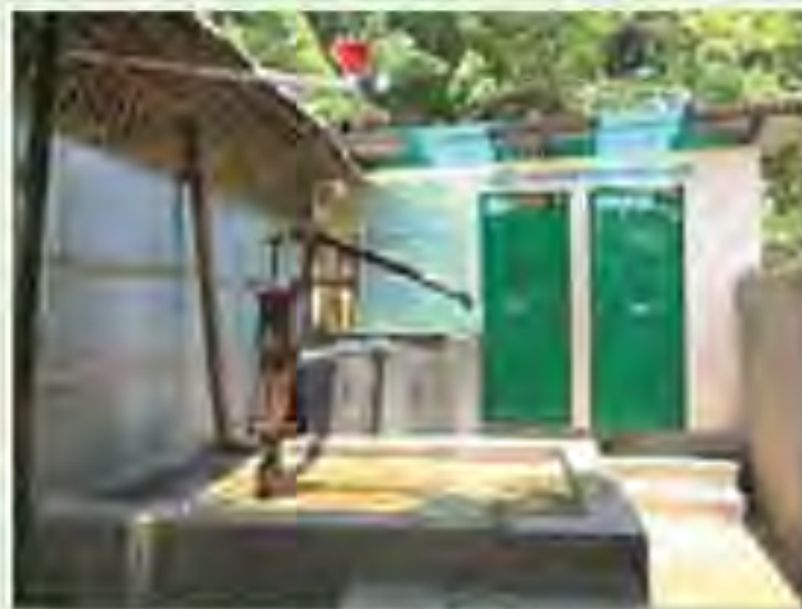
Water supply connected with DWASA and latrine chambers with septic tanks
