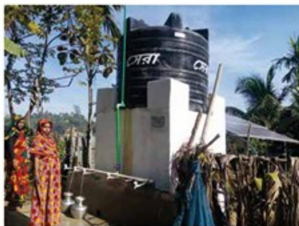
Submersible pump at Host community in Ukhiya.
